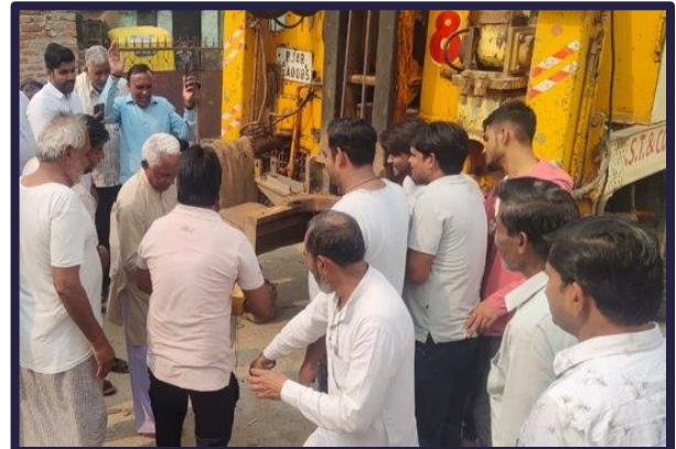
Borewell drilling at Kaluram Chowk
